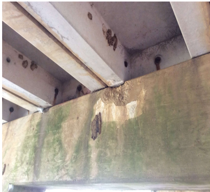
PHOTO 1 Description Intermediate substructure caps have shallow spalling in the bearing area under the units. Bent 2, Span 1 pictured.
