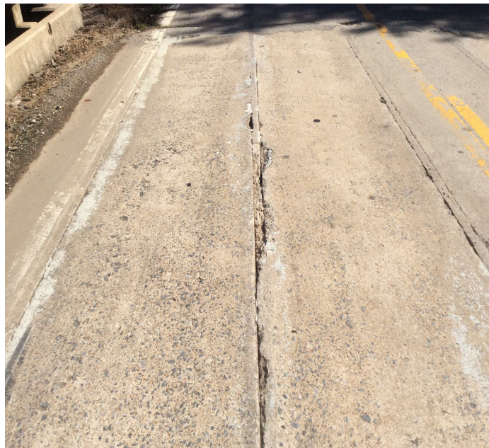
PHOTO 1 Description The grout joints between the units are deteriorating and appear to leak water on the superstructure and substructure. Span 4 at Units 2 & 3.
