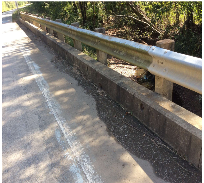
PHOTO 2 Description Dirt and debris along the gutters. Rt side pictured.
