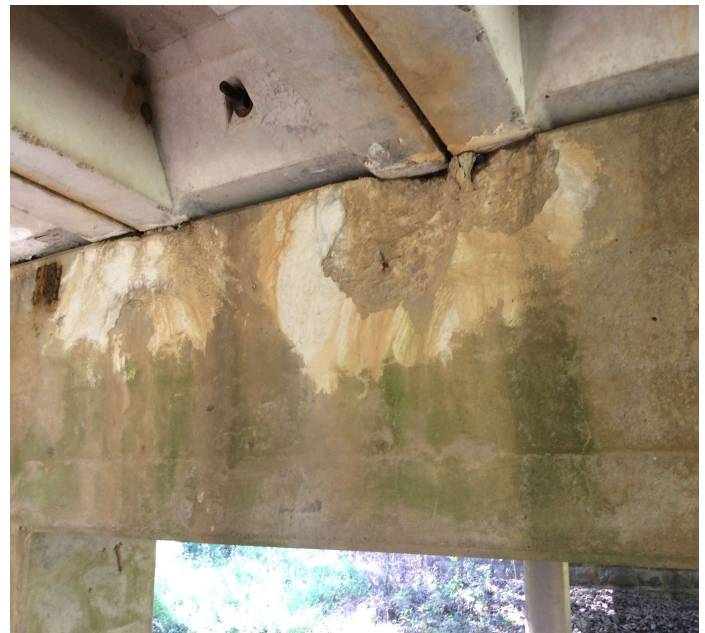
PHOTO 2 Description Intermediate substructure caps have shallow spalling in the bearing area under the units. Bent 3, Span 3 pictured.
