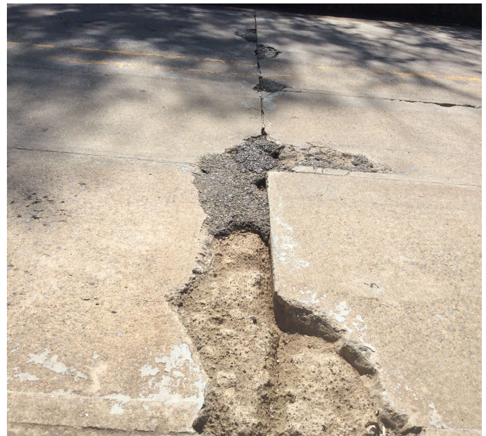
PHOTO 2 Description The concrete repairs over the intermediate bents is failing and causing potholes on the driving surface. Bent 2 pictured.
