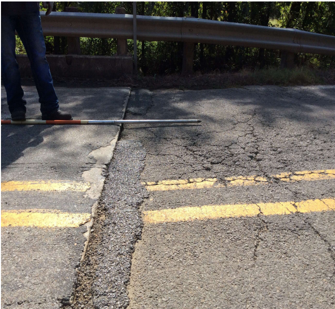
PHOTO 1 Description The asphalt approach roadway at both bridge ends has settled and has map cracking. Bent 1 pictured.
