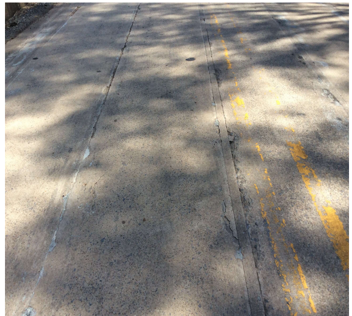
PHOTO 2 Description The grout joints between the units are deteriorating and appear to leak water on the superstructure and substructure. Span 2 at Units 2 & 3.
