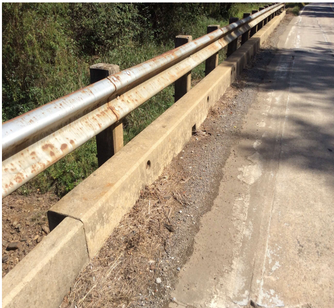
PHOTO 1 Description Dirt and debris along the gutters. Lt side pictured.
