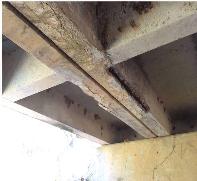
PHOTO 1 Description Spans 1 & 4 have longitudinal cracks, delaminated areas, and spalls with exposed reinforcing steel. Span 4, Unit 2 pictured.
