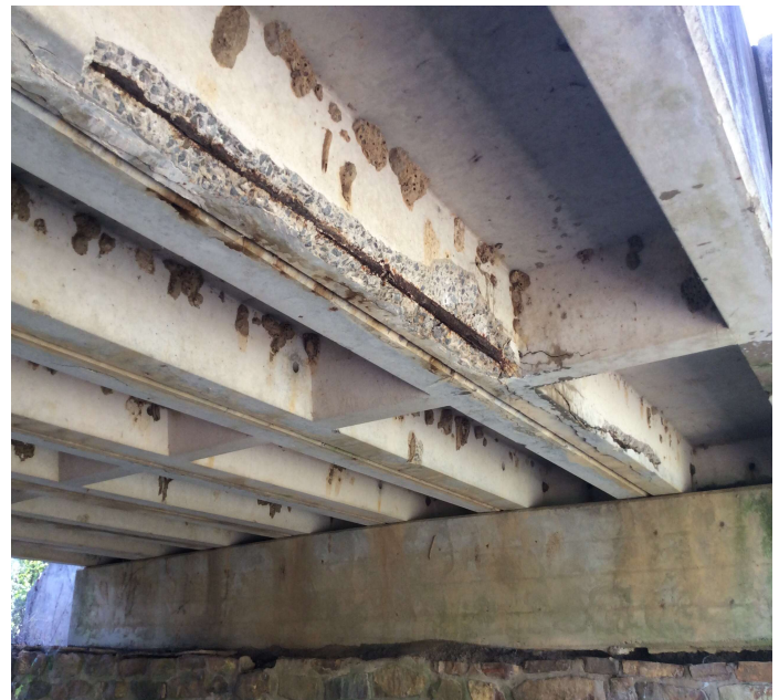
PHOTO 2 Description Spans 1 & 4 have longitudinal cracks, delaminated areas, and spalls with exposed reinforcing steel. Span 1, Unit 1 pictured.
