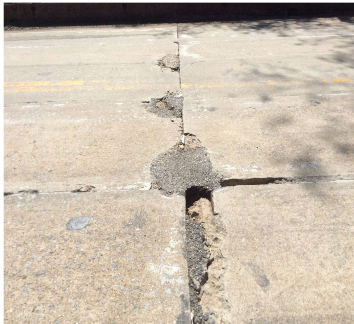
PHOTO 1 Description The concrete repairs over the intermediate bents is failing and causing potholes on the driving surface. Bent 4 pictured.
