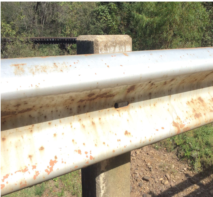
PHOTO 1 Description The Lt bridge railing is missing 2 anchor bolts at Span 1 and Span 3. Span 1, Post 4 pictured.
